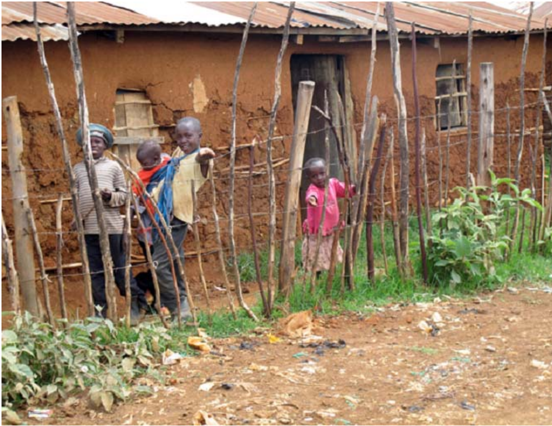
Picture 1. Typical housing and life in the Langas slums. Almost all houses are made of hardened mud and sticks, with iron sheet or tin rooftops.
